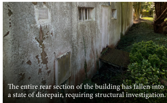
All brickwork is weathered and requires extensive work.
